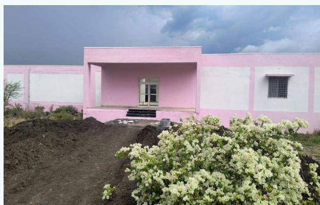
Construction of Library Room at College of Horticulture & Forestry Jhalawar
